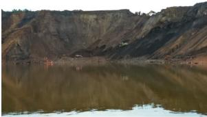
Prima facie cause of the accident: While a person was dozing muck at top of overburden dump which was over and above water logged pit, suddenly a portion of dump measuring abour 107 m (length) X 29.8 m (width) X 50 m (height) slithered and collapsed burying the operator deployed, he was recovered
